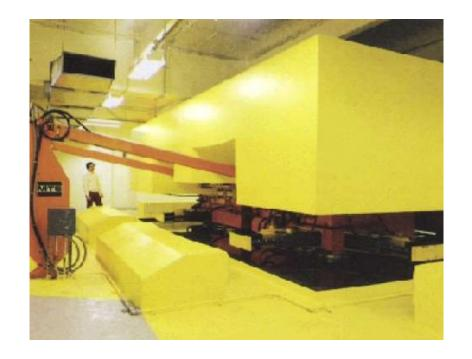
The weight is forced to oscillate at the same frequency as the building but 180 degrees out of phase.
